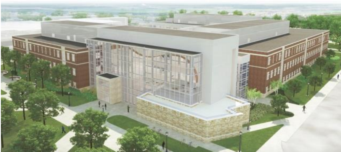
The 250,000 square foot MTSU Science building, open since 2014, is home to the Departments of Biology and Chemistry.
