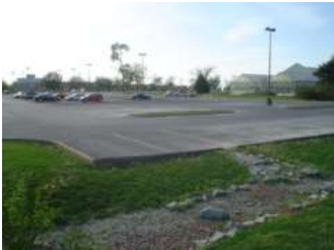
Figure 9: This is the inlet in relation to the parking lot that was mentioned in the above photos.
