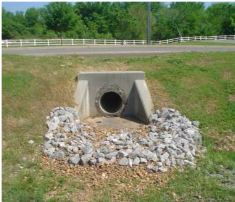
Figure 5 Culvert Post-remediation
