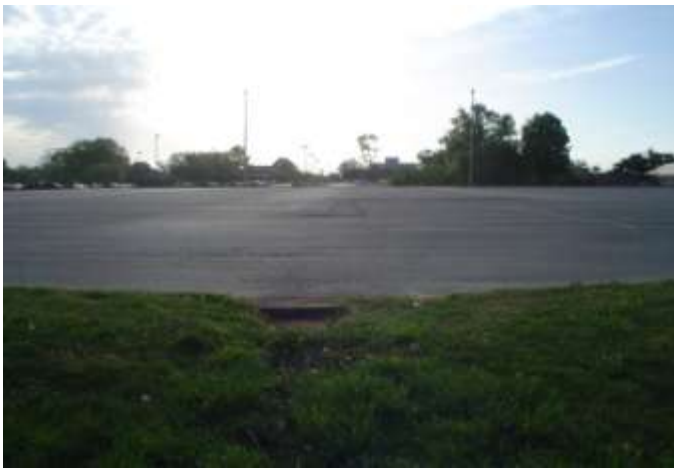
Figure 30: This is also facing against the flow to Raingarden #4.
