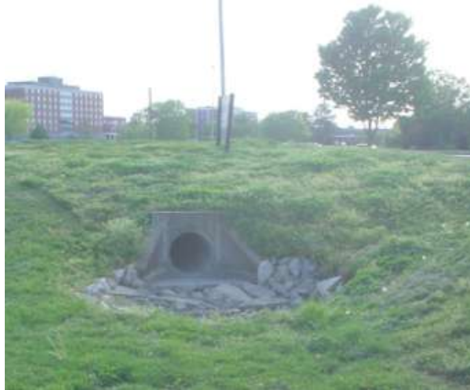
Figure 2 Culvert Pre-remediation
