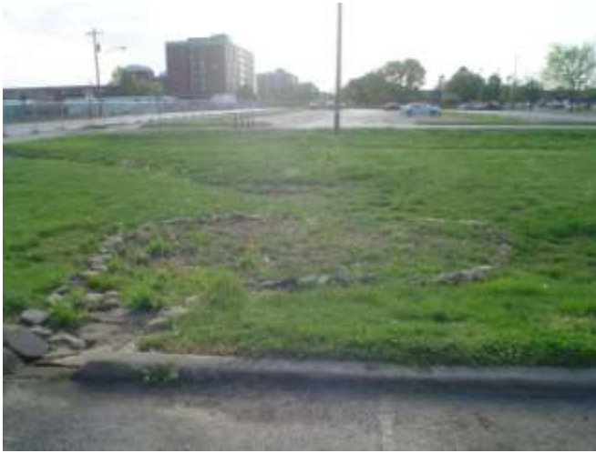
Figure 22: The inlet and Raingarden #3.
