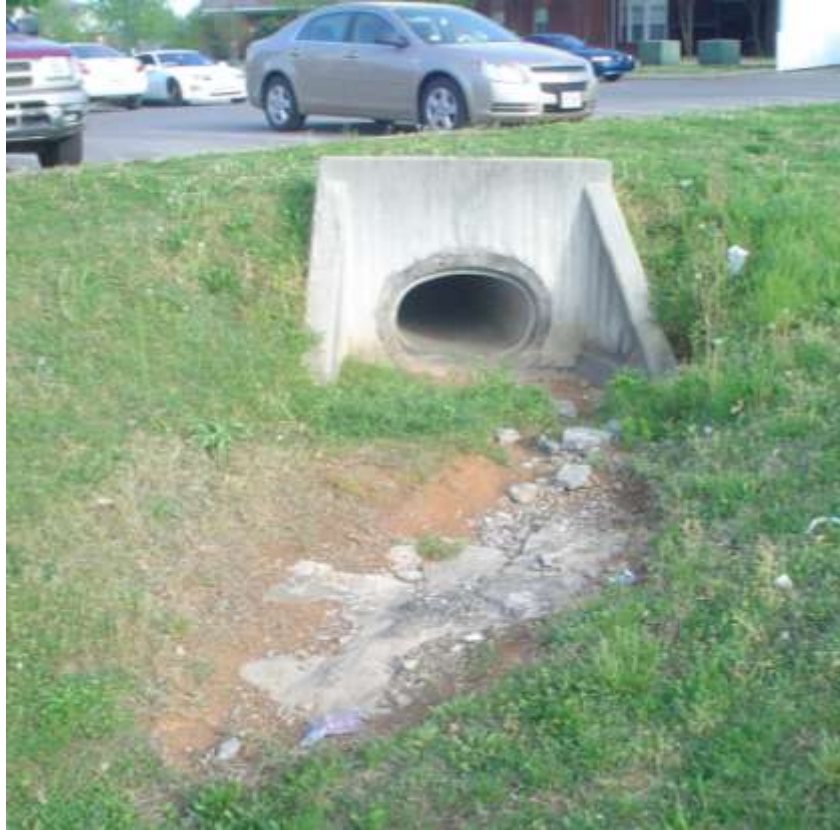
Figure 6 Inlet From Northwest Site to Southeast Site Pre-remediation
