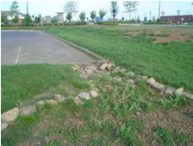
Figure 23: The inlet of Raingarden 3#.
