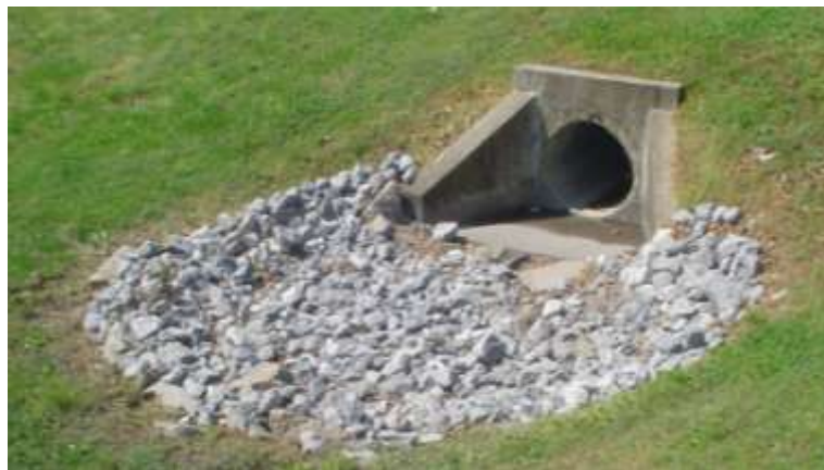
Figure 3 Culvert Post-remediation
