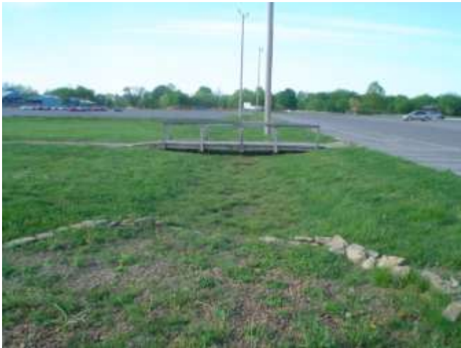
Figure 25: This photo is facing northward, which follows the flow of runoff towards Raingarden #3.
