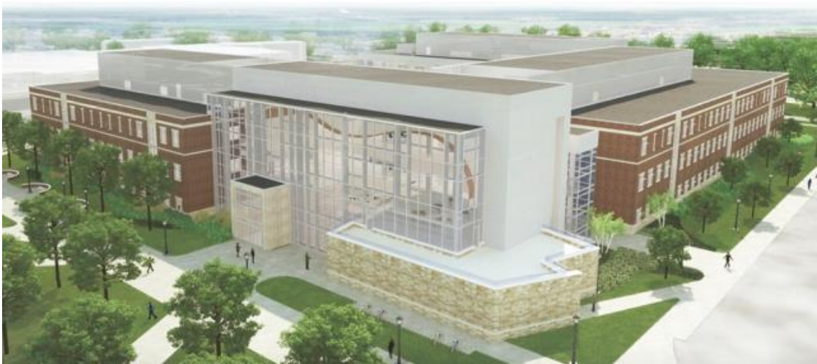
The new 250,000 square foot MTSU Science building opened in 2014, and is home to the Departments of Biology and Chemistry.
