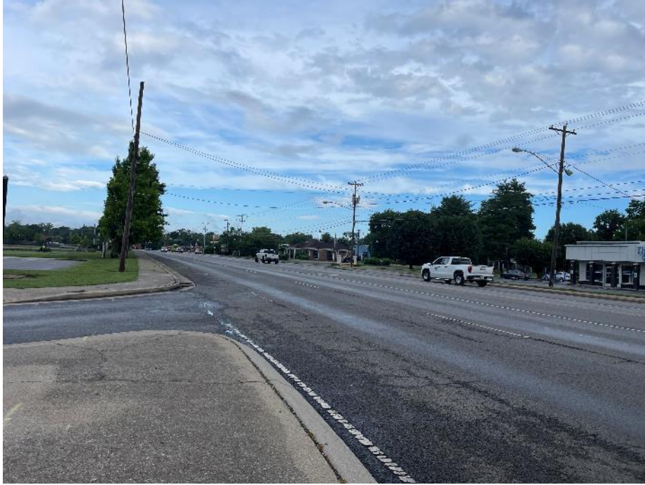
WEST VIEW ALONG GREENLAND DRIVE AT SITE #2
