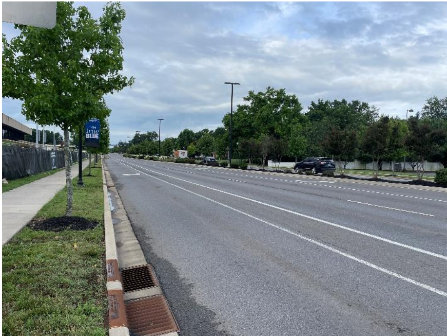
NORTH VIEW ALONG MIDDLE TENNESSEE BOULEVARD
