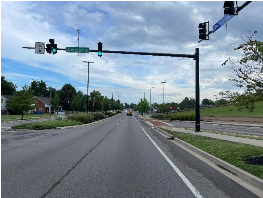
NORTH VIEW ALONG MIDDLE TENNESSEE BOULEVARD SOUTH OF SITES
